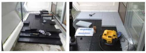
This balcony is raised approx. The floor is being raised and grey tiles are laid on top.
