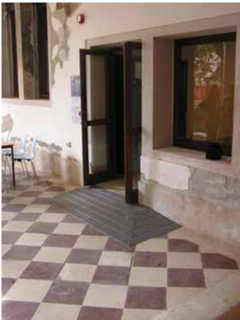
Custommade ramps for the UNESCO listed cemetery on the island of St. Michele. The ramps are adjusted to the building so that they will not do any damage.
