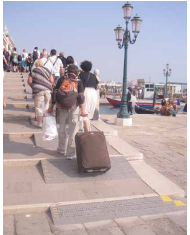
The ramps are installed at the bridge at the Marcus square in Venice, where 10.000.000 visitors yearly walk on the ramps.
