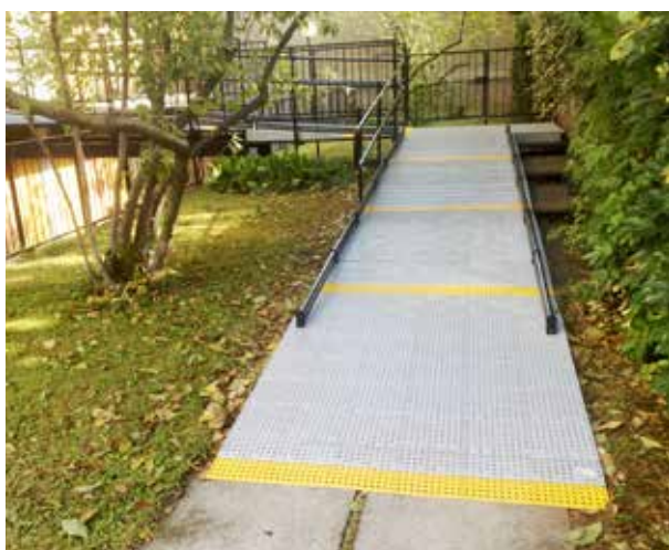
Custom made ramps with landings, rails and markings. Read more in our brochure Custommade ramps.
