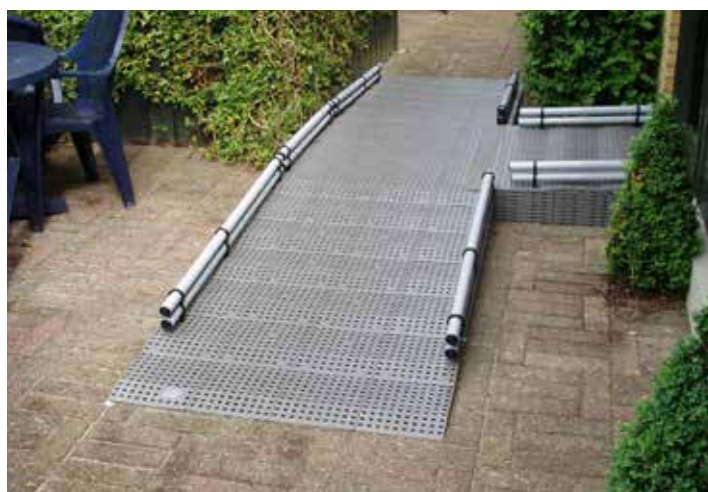
Ramp with platform, inclination 1:14 Good for manual wheelchairs.
