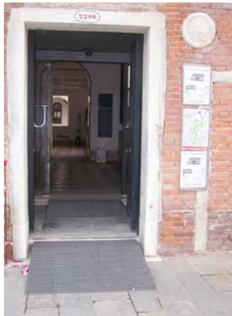
Custommade ramps for the UNESCO listed cemetery on the island of St. Michele. The ramps are adjusted to the building so that they will not do any damage.
