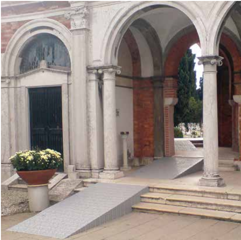
Custommade ramps for the UNESCO listed cemetery on the island of St. Michele. The ramps are adjusted to the building so that they will not do any damage.
