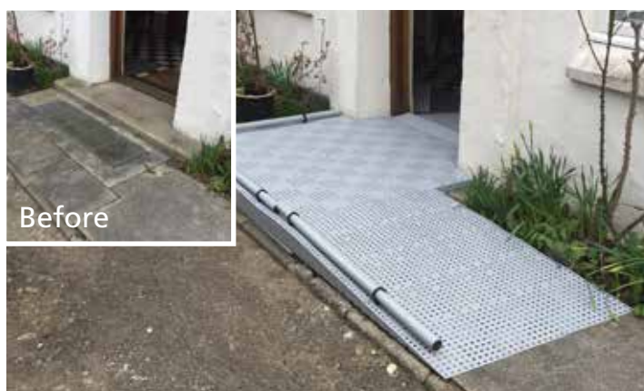
Ramp type II with platform inclination 1:14 Straight surface.
