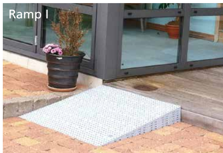
Ramp type I, inclination 1:7 Straight surface, good for electric wheelchairs.
