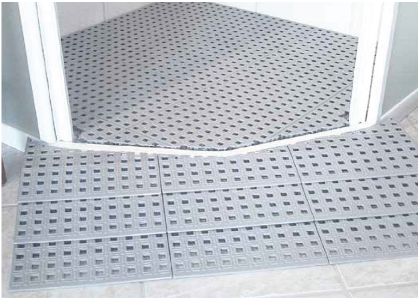
Example of a typical shower unit. A shower tray like this one will be filled up with tiles and if necessary fitted with a small ramp.
